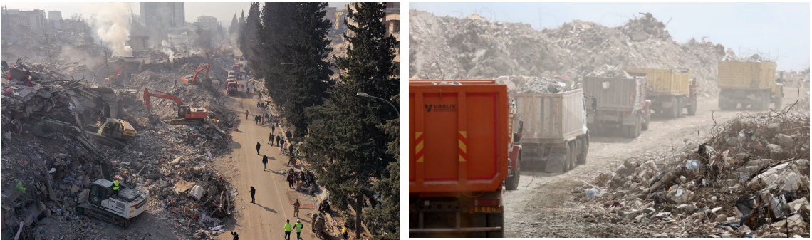
Fig. 6. Debris removal works after the earthquake in the region [35, 36]
